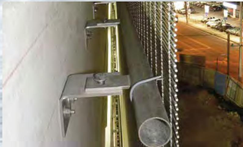
Intermediate mounting: round tube and wire connectors.
